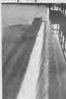
WATER OUTLET or sewer allows a thin film of water over its edge to provide a slight movement in the primary separator. This allows oil to float to the top where it can be skimmed off.
